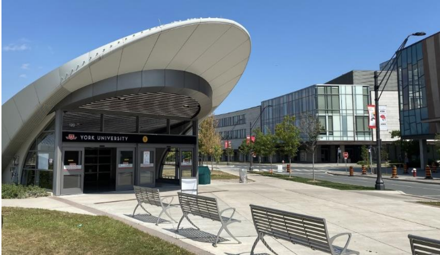
York University Subway Station
