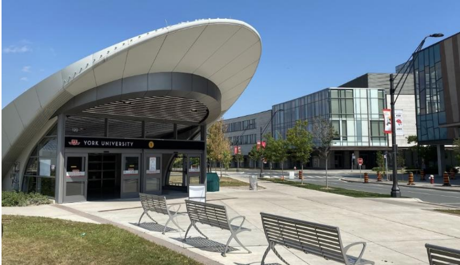
York University Subway Station
